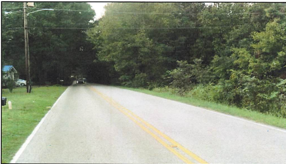
35 Railroad Avenue STREET SCENE - NORTH VIEW
