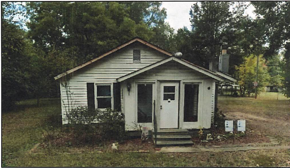
35 Railroad Avenue FRONT VIEW
