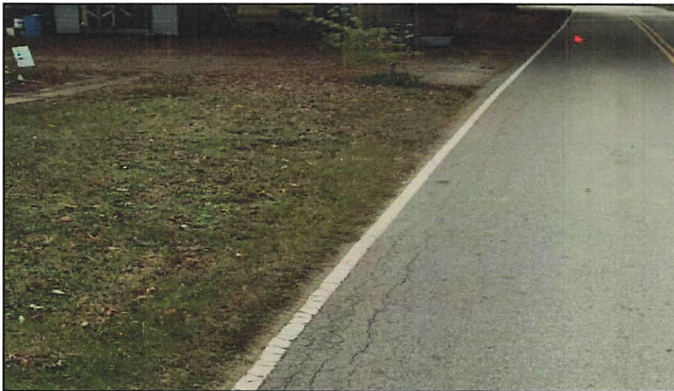
35 Railroad Avenue ACQUISITION AREA ON LEFT
